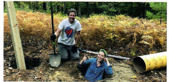
Peter Hubbard & Sami Wolf building our new kiosk.
